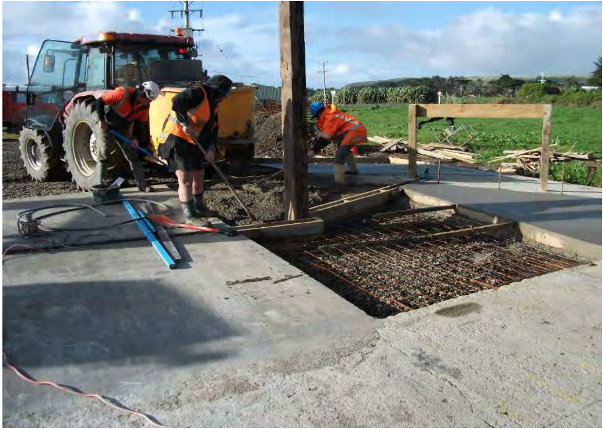
New Workshop Wash Down Being Constructed
