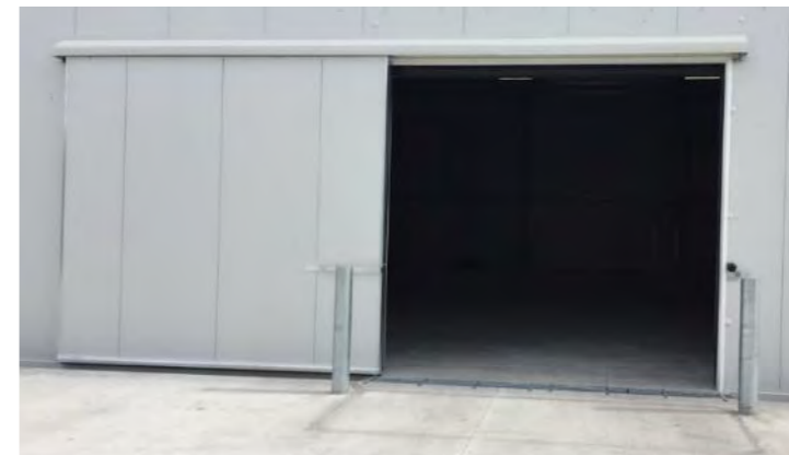
Coldstore sliding Door
