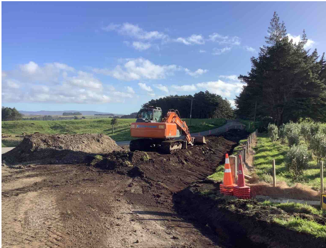
WW-0/Te Matarae Intersection Works
