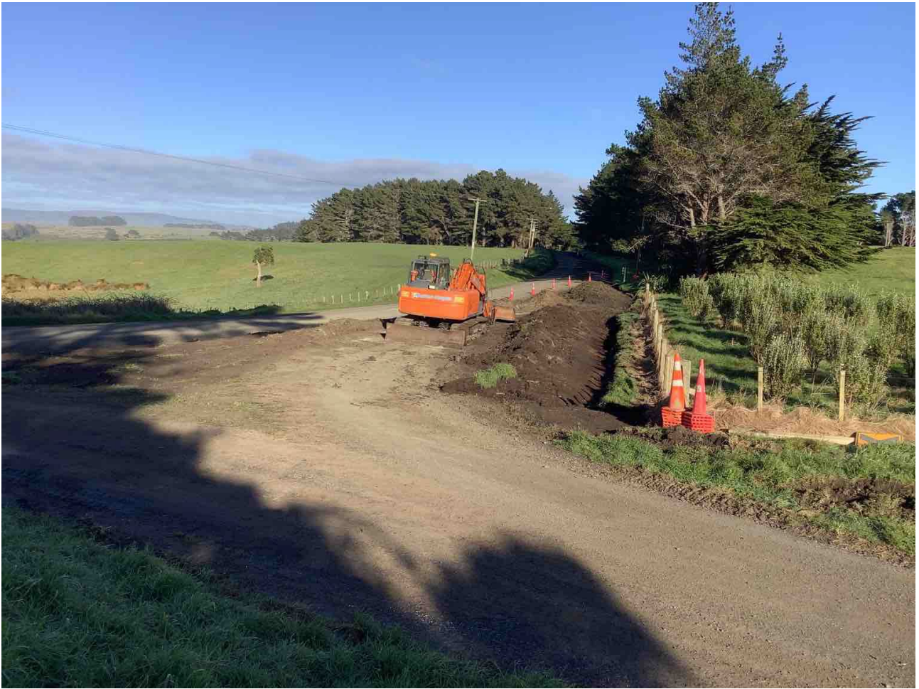
WW-O/Te Matarae Intersection Works
