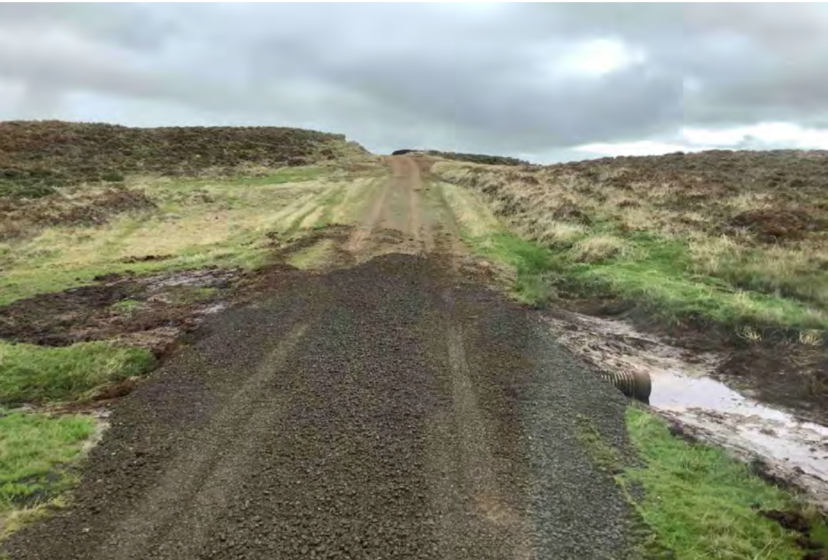
Tuku Road Culvert Replacements
