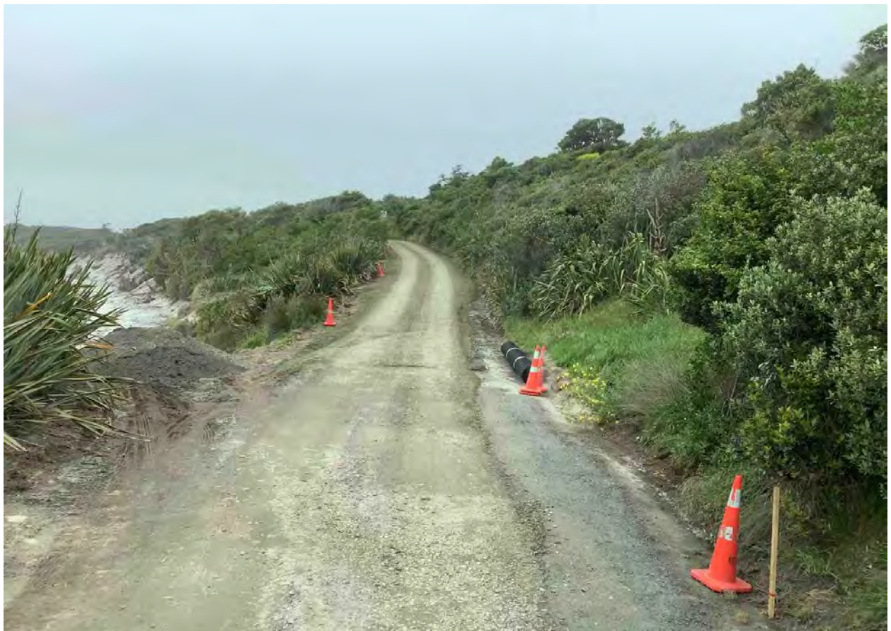
Kaingaroa Rehab Works
