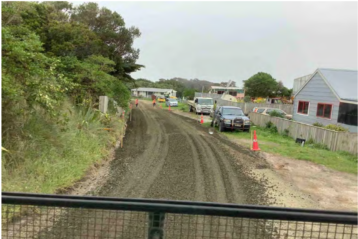
Kaingaroa Rehab Works
