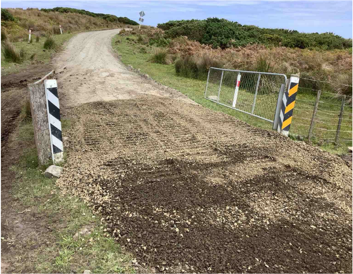
Damaged Cattle Stop Removed For Repairs
