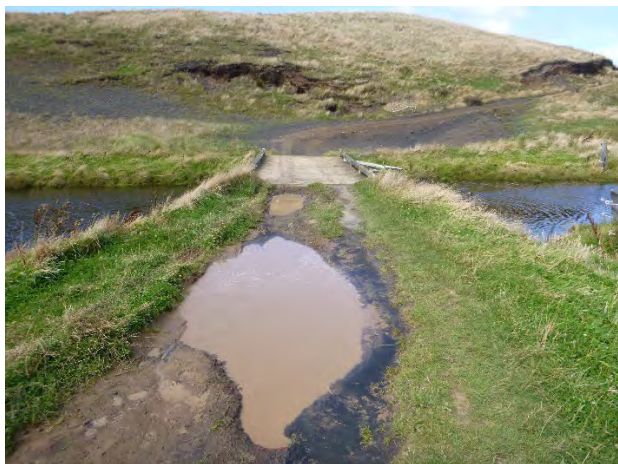
Figure 4-17: Waipaua (#P2) approach potholes
