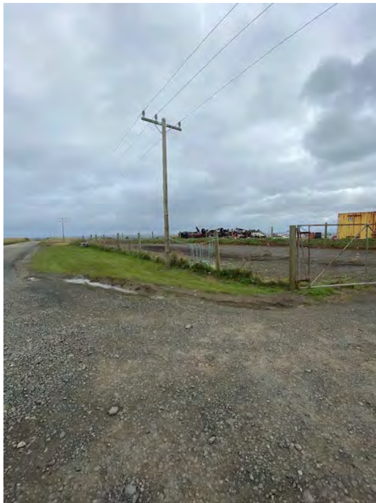
Remodelled front face of the Te One Transfer Station
