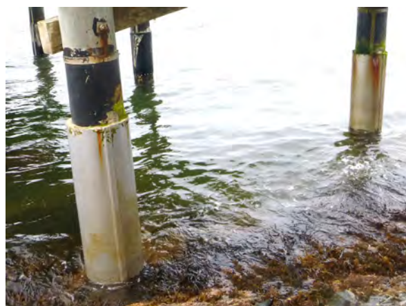
Figure 3-13: Owenga pile s/steel reclad
