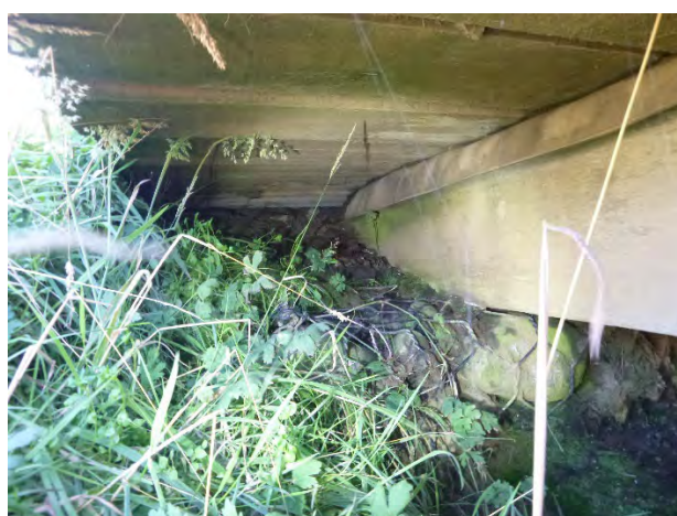
Figure 4-4: North Head (#P3) no backing boards
