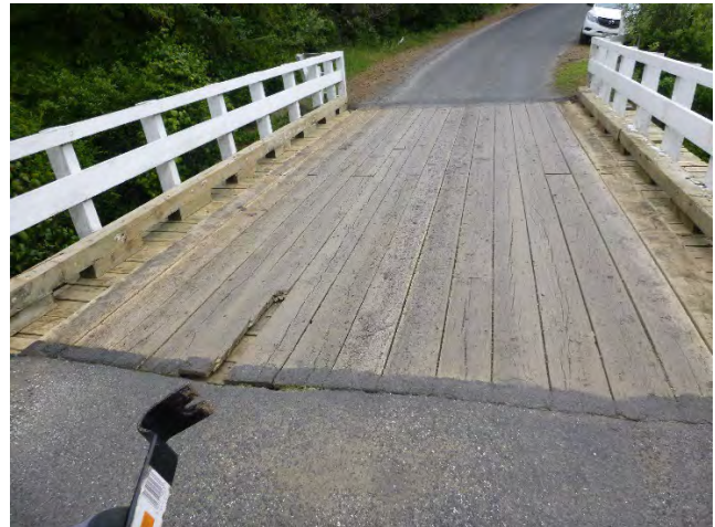
Figure 4-10: Hawaiki (#19) loose running boards
