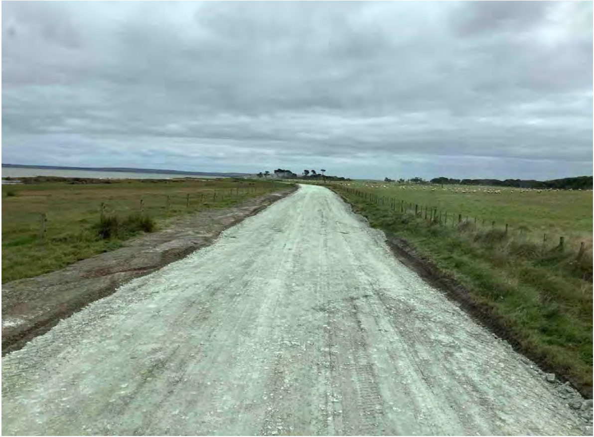
North Road Strengthening Works
