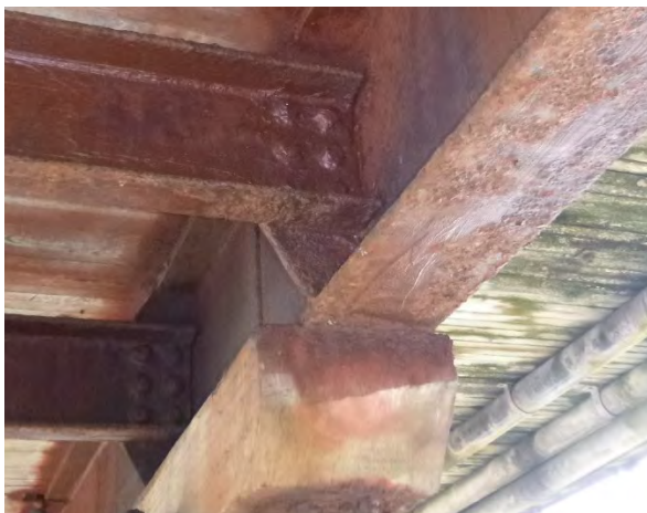
Figure 3-1: Lower Nairn (#20) Goldseal failing from the 2021 inspection
