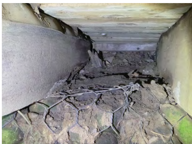
Figure 4-3: North Head (#P3) no backing boards
