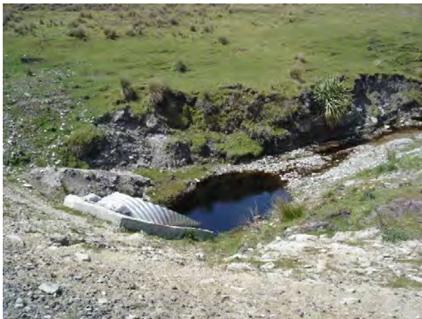
Figure 4-13: Whangatete (#1) typical scour hole at outlet
