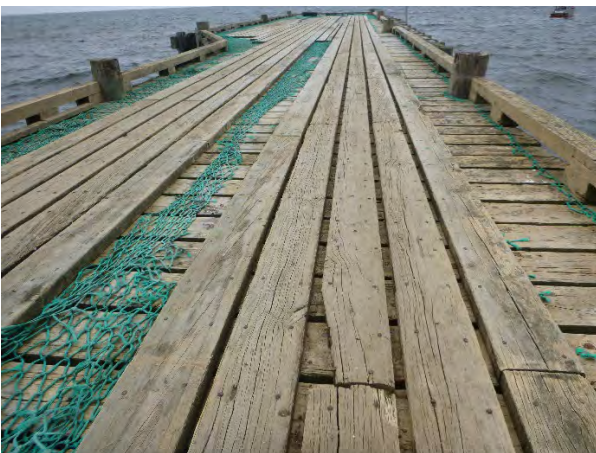
Figure 3-8: Owenga water blasted deck
