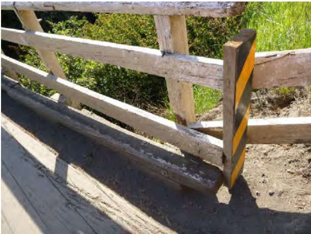
Figure 4-11: Te Awainanga (#15) handrails in 2015, before painting in 2016
