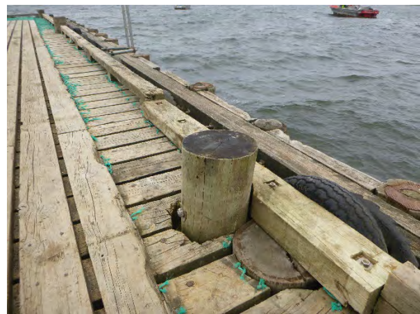
Figure 3-9: Owenga repaired bollard pile
