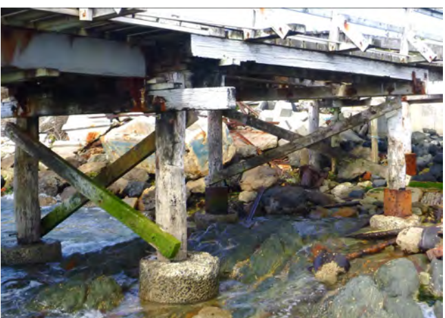
Figure 3-17: Kaingaroa upgraded piles
