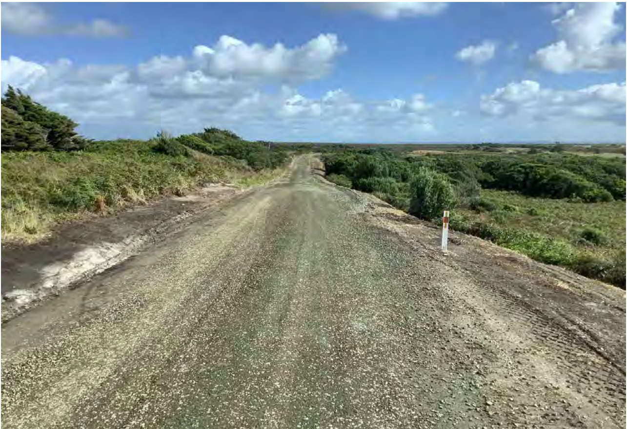
High Shoulder Removal At Matarakau
