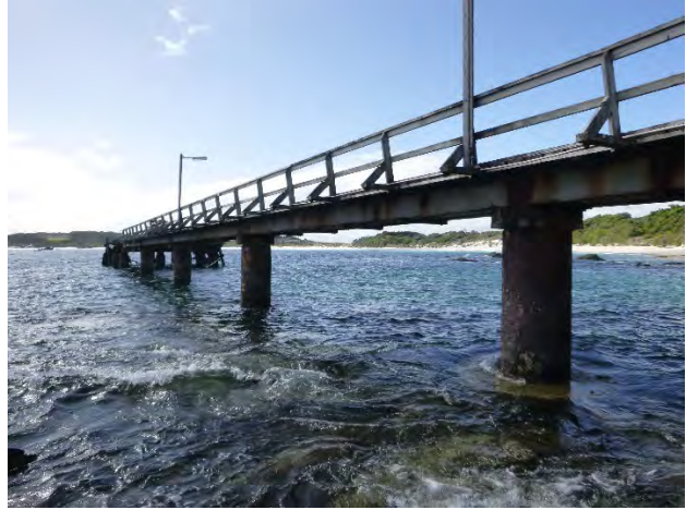
Figure 3-21: Kaingaroa repaired handrail
