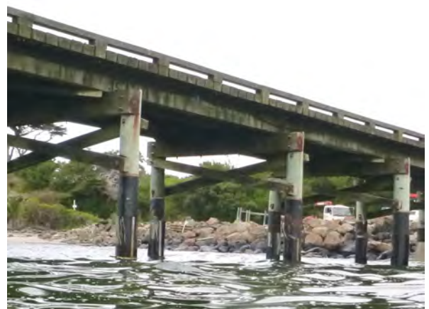
Figure 3-11: Owenga lift bracing and PE reclad
