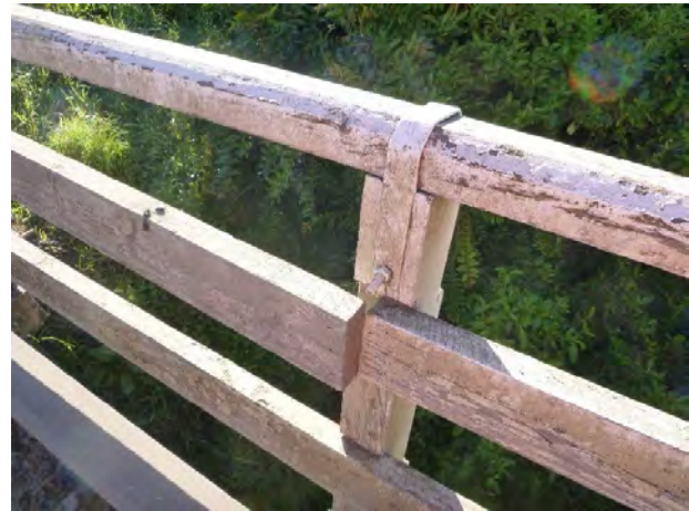
Figure 4-12: Te Awainanga (#15) handrails in 2017, after painting in 2016
