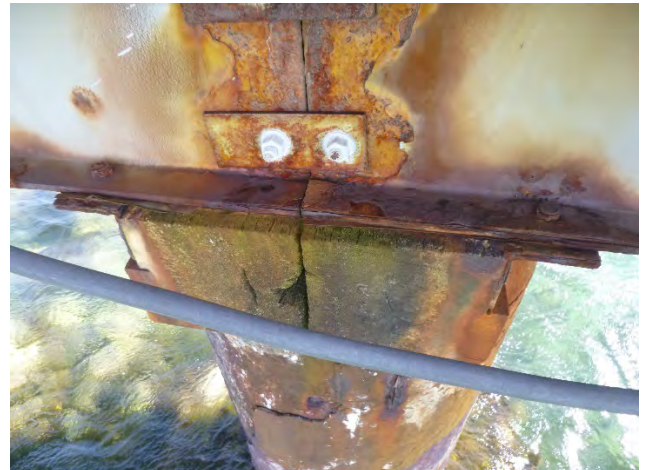
Figure 3-19: Kaingaroa upgraded HD fixings
