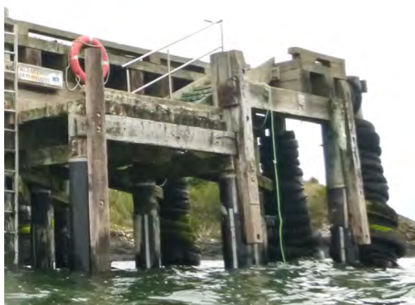
Figure 3-12: Owenga launch platform repaired
