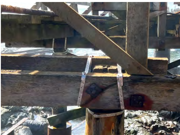
Figure 3-18: Kaingaroa upgraded timber fixings
