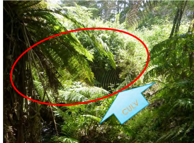
Figure 4-16: Awatotara (#11) waterway clearance required
