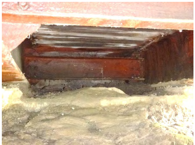
Figure 3-29: Te Awainanga debris on TR abutment
