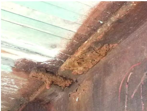
Figure 3-2: Lower Nairn (#20) Goldseal failing from the 2023 inspection
