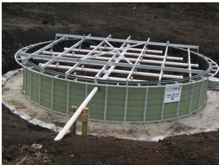
Figure 3-3: Completed leachate treatment plant.
