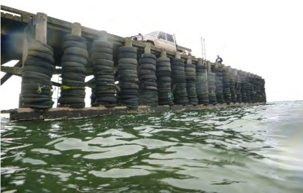
Figure 3-10: Owenga additional tyres on fender
