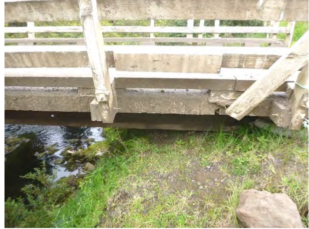
Figure 4-6: Te Awainanga (#15) debris on bearing shelf
