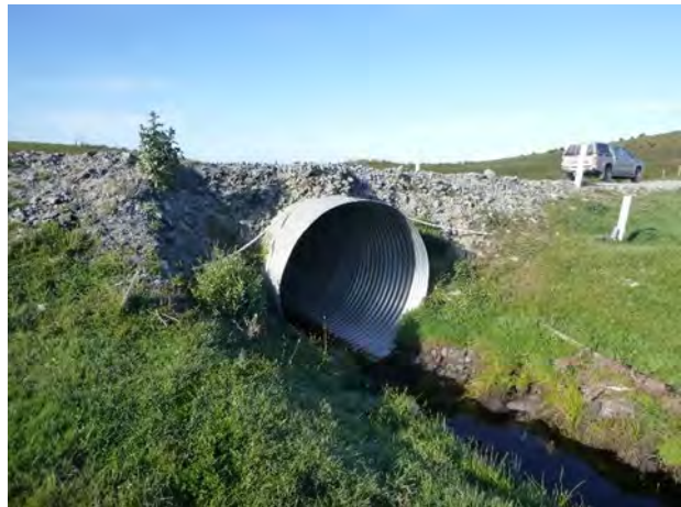
Figure 1-2: Waikawa Culvert (#23) – Port Hutt Road
