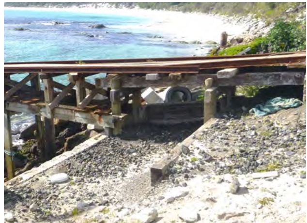
Figure 3-15: Kaingaroa upgraded ramp support
